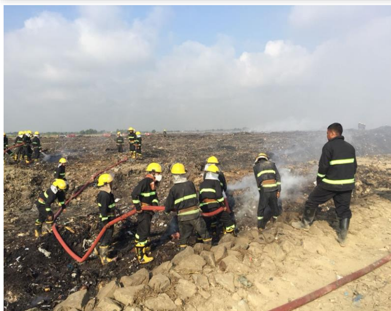
Fire Service Department of Myanmar doing excavation in Zone A of Htein Pin Dump Site to extinguish the deep-sited fire under the garbage that being piled up for nearly 2 decades.
