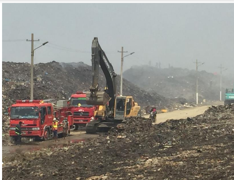
Fire Service Department of Myanmar doing excavation in Zone A of Htein Pin Dump Site to extinguish the deep-sited fire under the garbage that being piled up for nearly 2 decades.
